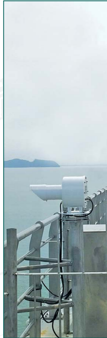
MEL 250L Penang Bridge - MALAYSIA
